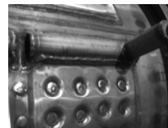
Typical Half-Pipe Header
